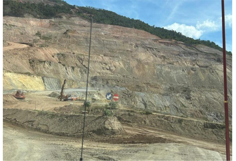
Figure 10. Open-pit area during ongoing pushback activities
