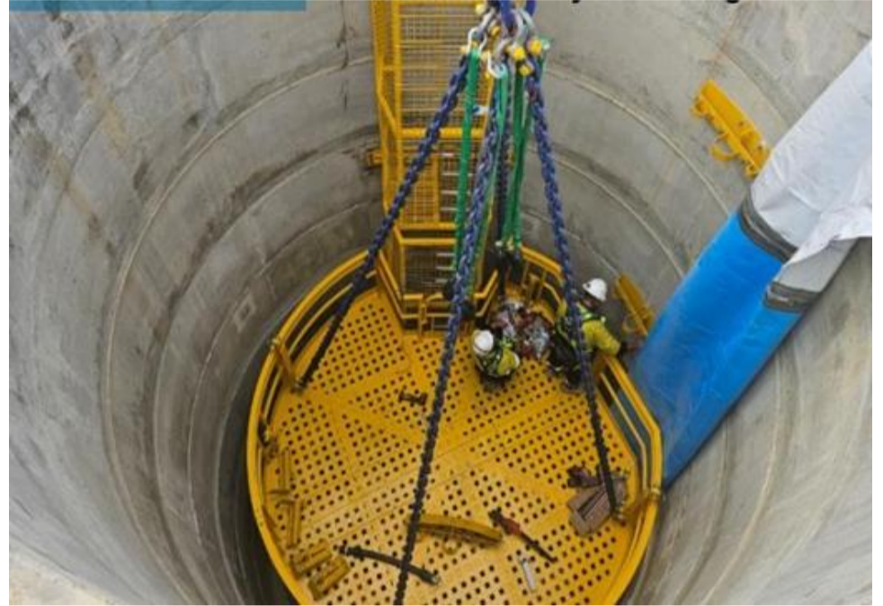
Figure 16. Shaft Sink Construction (Single Deck Stage)
