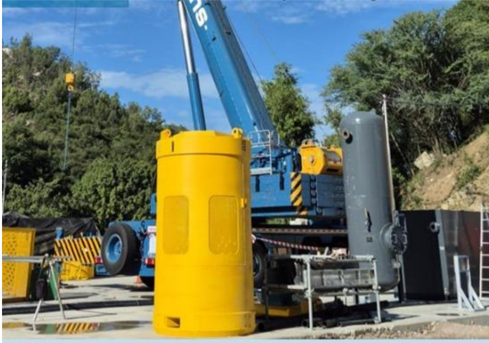
Figure 15. Shaft Sink Construction (Equipment Kibble)
