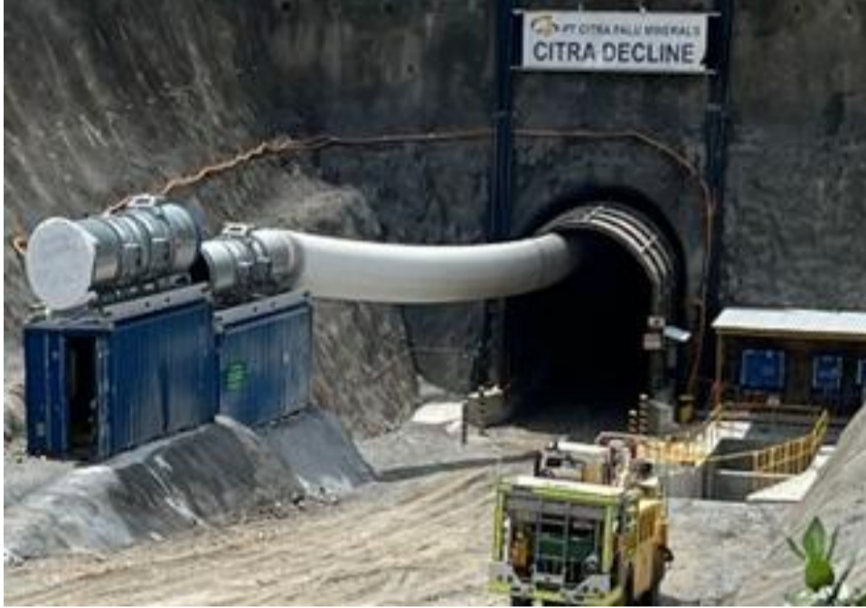
Figure 12. Portal to the underground mine tunnel
