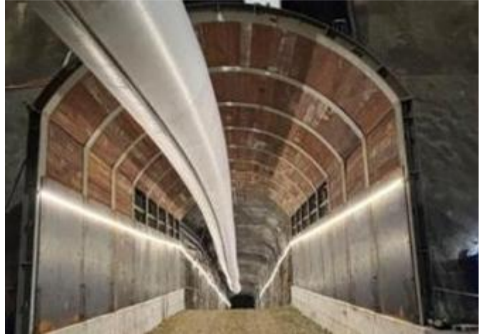
Figure 13. Underground tunnel (decline)
