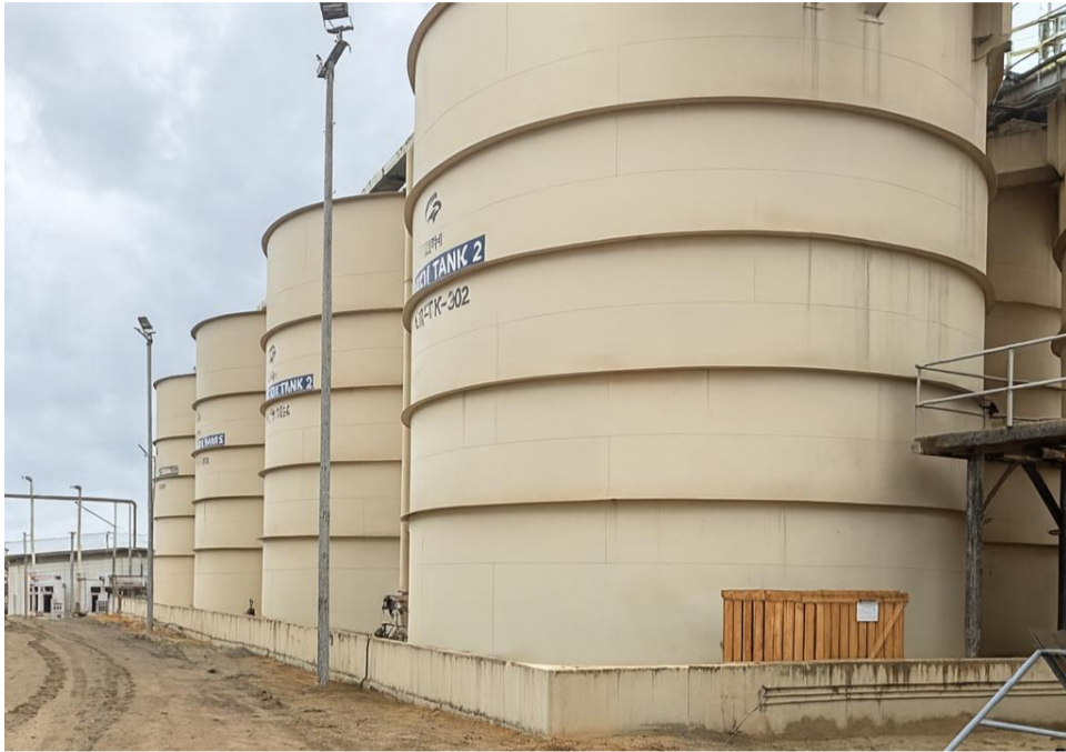
Figure 5. Carbon-in-leach tanks to extract gold and silver using cyanide
